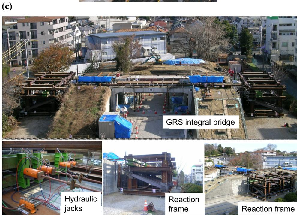
Fig. 7. A full-scale model of GRS integral bridge constructed at Railway Technical Research Institute: (a) overall structure (Suga et al., 2012); (b) the left side abutment in Fig. a under construction (27 November 2008); and (c) full-scale loading test (January 2012) (Koda et al., 2013).
