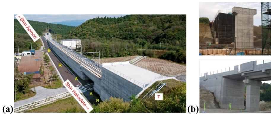
**Fig. 3.** (a) A view of a variety of GRS structures at Mantaro section of the south part of Hokkaido Shinkansen; and (b) GRS bridge abutment (13.4 m-high) during and after construction, near Mantaro tunnel.
